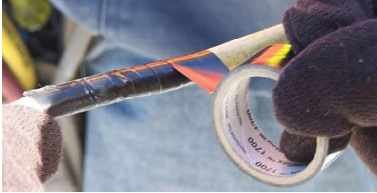
Electrical tape is not an approved repair method for damaged cords.
